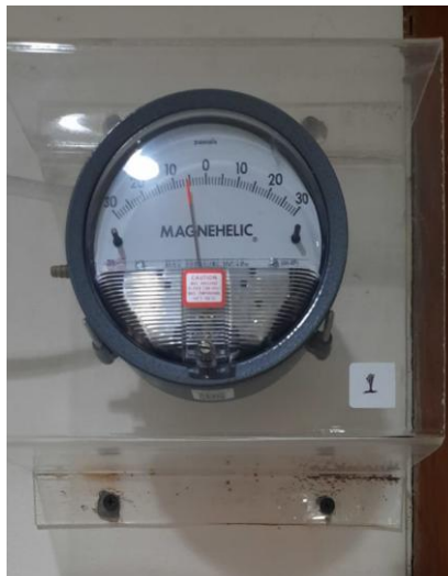
Gambar 6. 7. Magnehelic Kamar isolasi, Tekanan -5 Pascal
