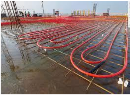
Gambar 6. 1. Thermally active building systems (TABS)
