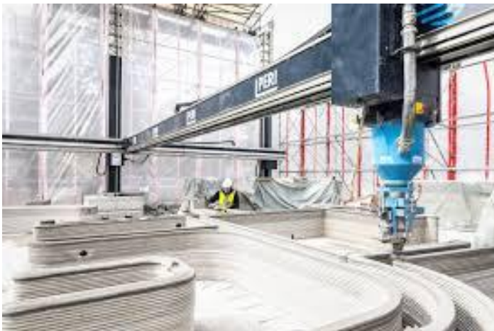
Gambar 7. 14. 3D Printing Bangunan
